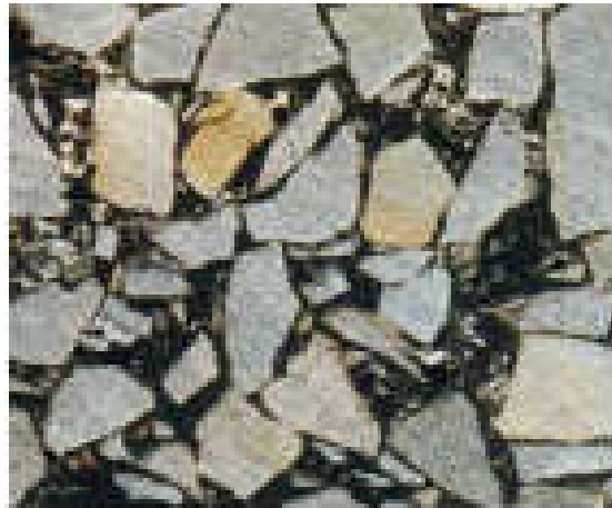
(a) Stone Matrix Asphalt
