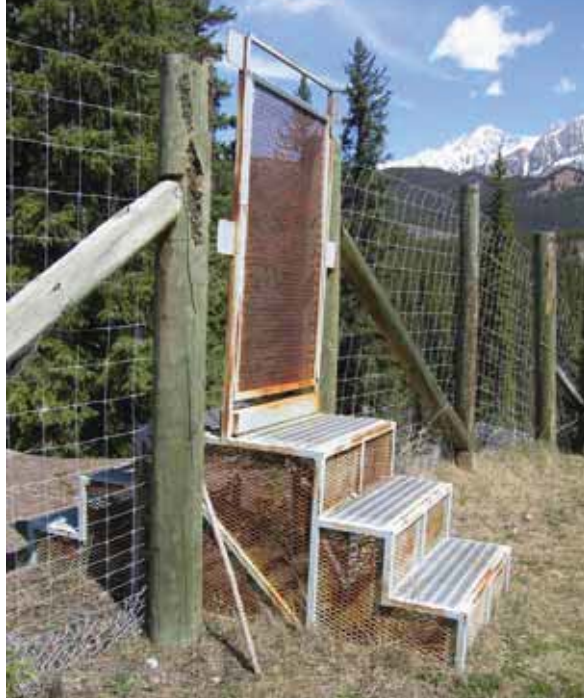
Figure 54. Photo. Swing gate in fence (spring loaded) allowing access for people, along the Trans-Canada Highway in Banff National Park, Alberta, Canada (copyright: Adam Ford, TCH research project/WTI-MSU).
