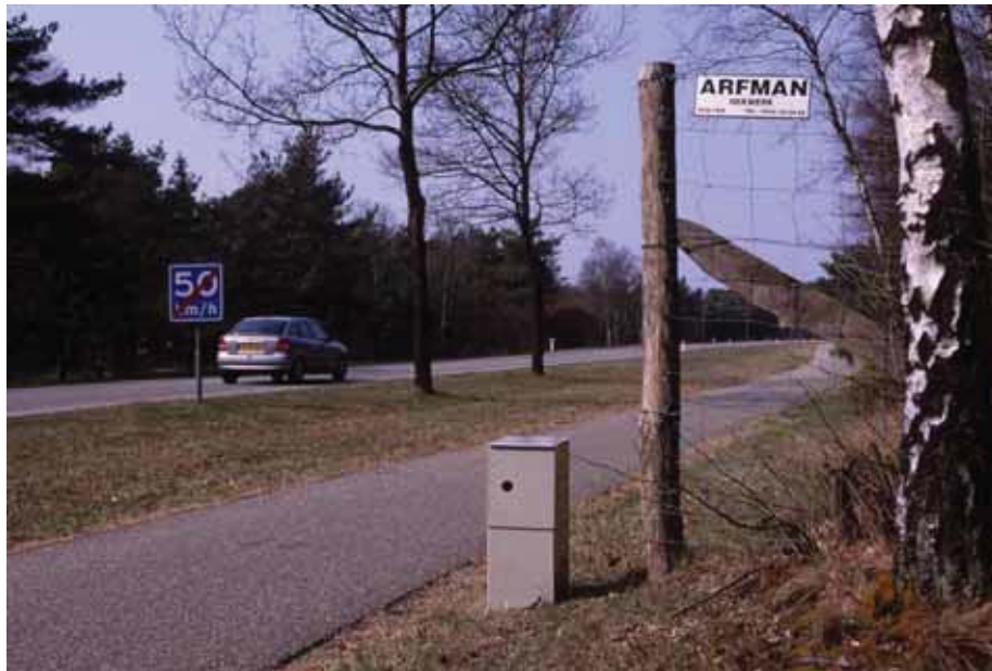
Figure 44. Photo. Gap in a wildlife fence combined with an animal detection system, wildlife warning signs, and advisory speed limit reduction, The Netherlands (copyright: Marcel Huijser).
