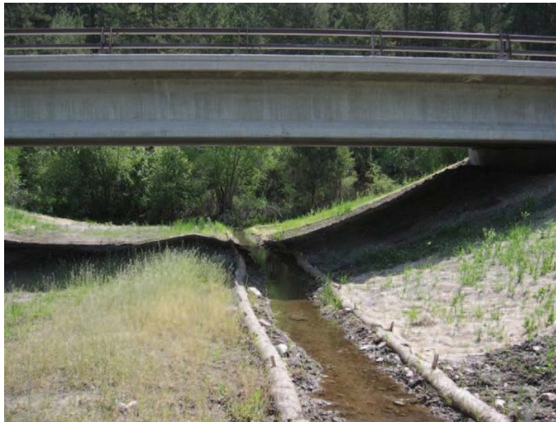
Figure 58. Photo. Long bridges do not have to be excessively large to provide ample space for wildlife crossings. While not exceedingly long, this bridge provides plentiful space for both the stream and wildlife to cross.
