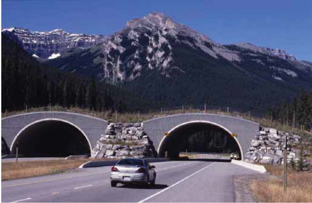
Figure 46. Photo. Wildlife overpass in Banff National Park, Alberta, Canada (copyright: Marcel Huijser).
