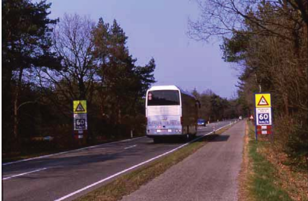
Figure 43. Photo. Gap in a wildlife fence accompanied by wildlife warning signs and advisory speed limit reduction, The Netherlands (copyright: Marcel Huijser).
