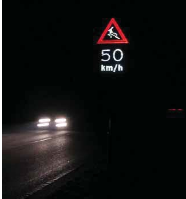
Figure ES4. Photo. Wildlife warning and advisory speed limit reduction signs triggered by an animal detection system in ‘t Harde, The Netherlands (copyright: Marcel Huijser).
