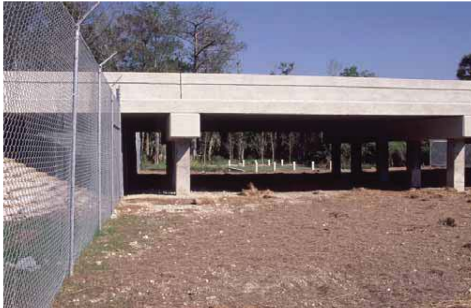
Figure 47. Photo. Underpass in southern Florida that allows for ecosystem processes (hydrology) as well as wildlife use, including the Florida panther (copyright: Marcel Huijser).
