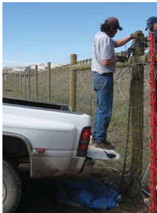
Figure ES13. Photo. Wildlife fencing along Interstate 90 near Bozeman, MT (copyright: Marcel Huijser).
