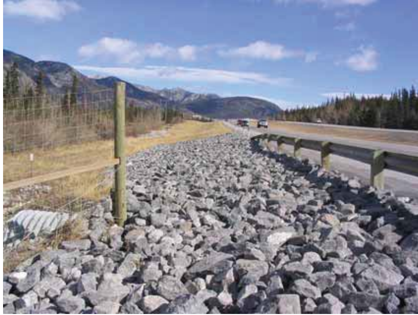
Figure 51. Photo. The boulder field at the fence end at Dead Man’s Flats along the Trans-Canada Highway east of Canmore, Alberta, Canada (copyright: Bruce Leeson).
