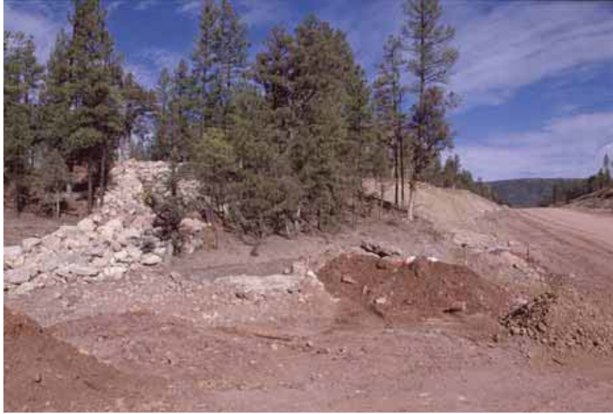
Figure 56. Photo. Large boulders placed in the right of way as a barrier to elk and deer with a view of State Route 260 (under construction) in Arizona (copyright: Marcel Huijser).
