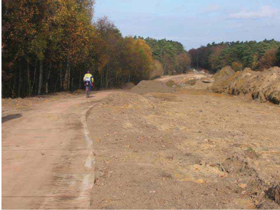
Figure 59. Photo. Road removal in progress in Belgium (note that a path for pedestrians and bicyclists remains in place.) (copyright: Bethanie Walder).
