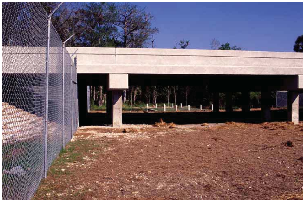
Figure ES14. Photo. Wildlife underpass in southern Florida that allows for ecosystem process (hydrology) as well as wildlife use, including the Florida panther (copyright: Marcel Huijser).
