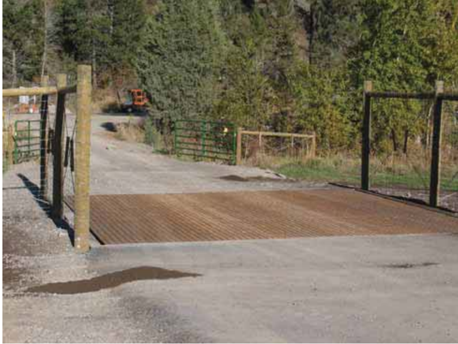
Figure 52. Photo. Wildlife guard along U.S. Highway 93 on the Flathead Indian Reservation, MT (copyright: Marcel Huijser, WTI).
