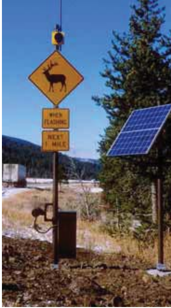
Figure ES19. Photo. Animal detection system along U.S. Highway 191 in Yellowstone National Park, MT (copyright: Marcel Huijser).
