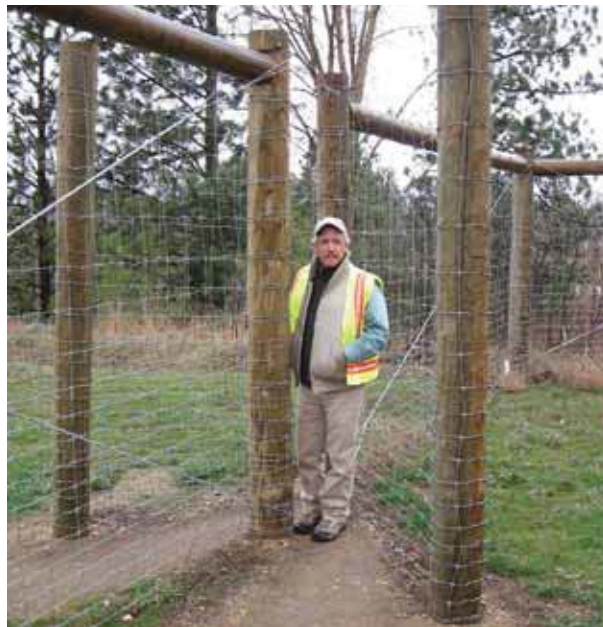
Figure 53. Photo. Angled opening in fence allowing access for people along U.S. Highway 93, MT (copyright: Marcel Huijser, WTI).
