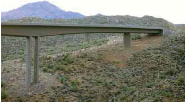
Figure ES16. Photo. Long bridge on Arizona Highway 260 constructed in such a way as to minimize the impact to soil and vegetation (copyright: Marcel Huijser).
